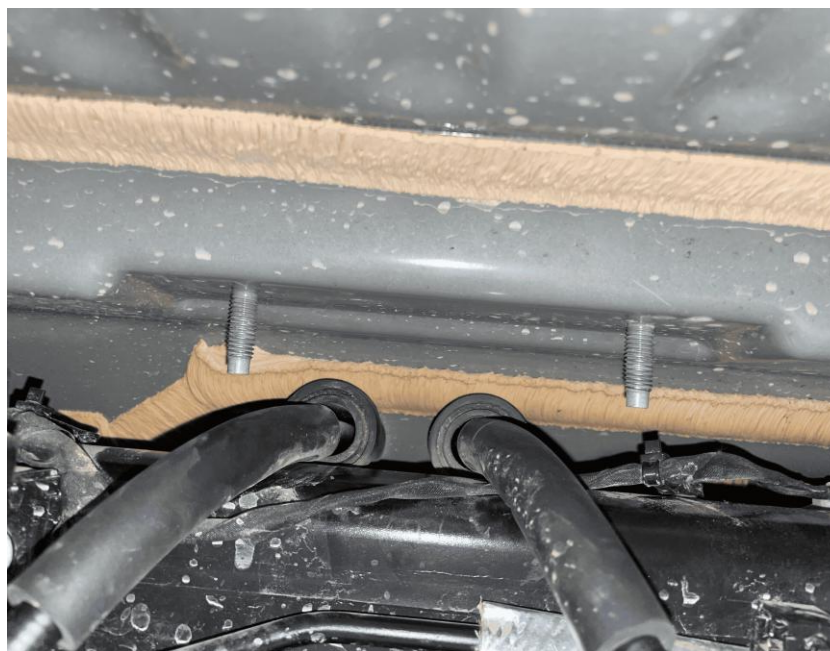
Figure 23: Emergency cable bracket removed
